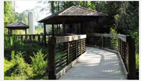
TOWN CREEK PARK WALKING TRAIL
